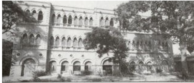
Building in Nursing Mess area part of the original Civil Hospital Karachi since its inception.
