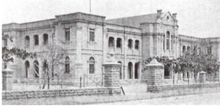
Bai Virbaiji Anglo Vernacular High School - Building commissioned in 1906
