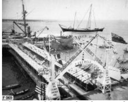
Farewell arch erected by the Karachi Port for the Royal visit of King George V in 1906
